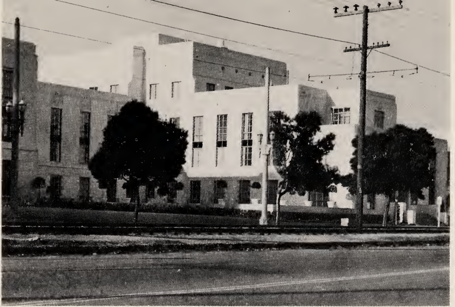
ABOVE: Thalberg Building, Metro-Goldwyn-Mayer lot, Culver City, where Huxley, Loos, and Isherwood wrote in the mid-1930s. (Photograph by Bob Plunkett. Courtesy of Jim Heimann.)
